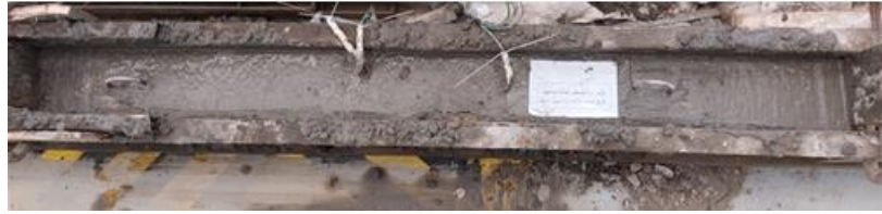
FIGURE 2. Typical beam preparation and casting.
